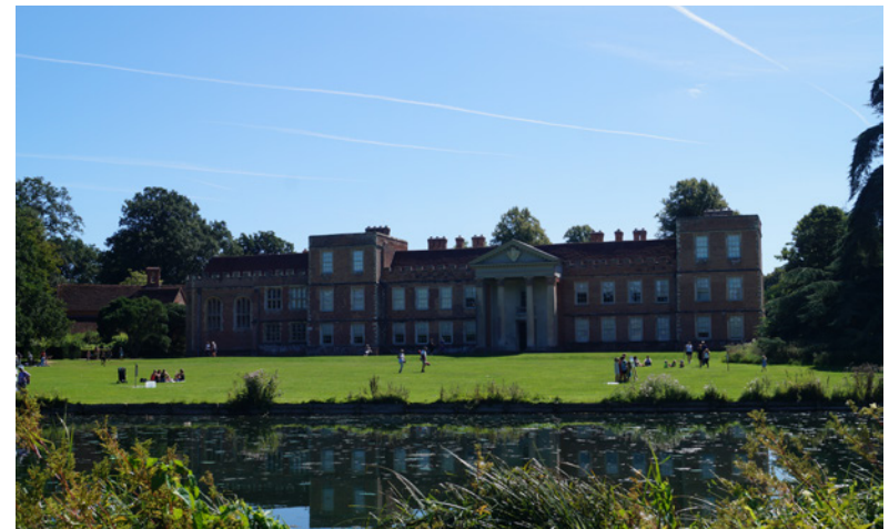
Figure 16: The Vyne, Grade I listed house
