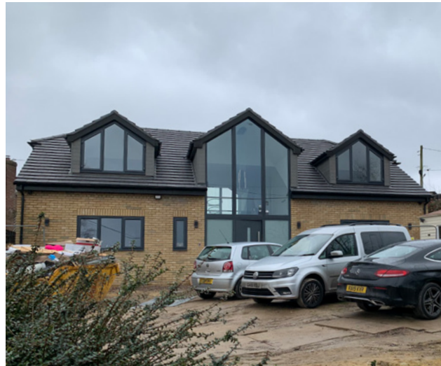
Figure 33: A new, contemporary style house with some elements that are in keeping with the historic character, such as gabled dormers and the low scale. The sand brick and extensive glazing is out of character.
