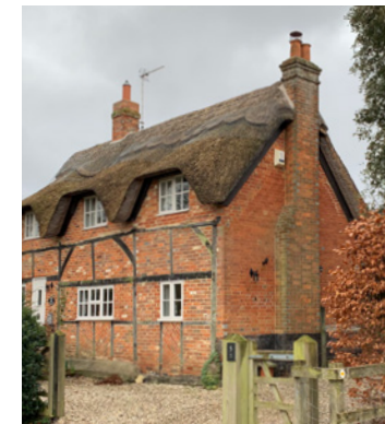
Figure 106: Thatched roof, red brick, black exposed timber frame
