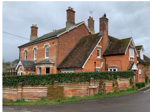
Figure 60: A large, detached, corner dwelling on Vyne Road with a steep, varied roofline with feature chimneys, which creates a noticeable landmark.
