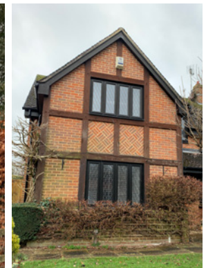
Figure 107: Red brick front, exposed timber frame
