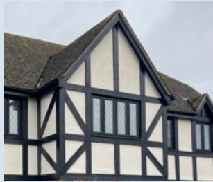
Exposed timber framework
