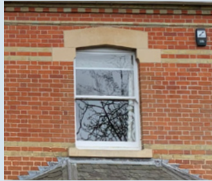
Sash window and fenestration detail
