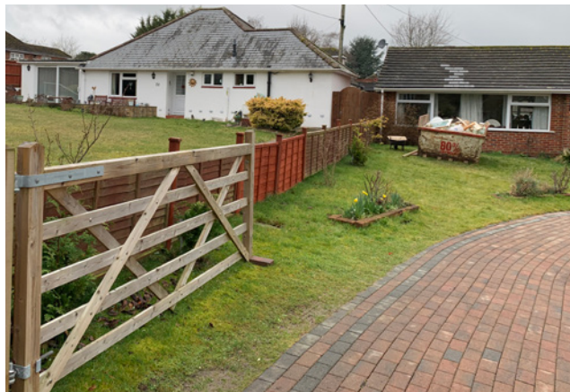
Figure 35: Bungalows with large front gardens which create an open, spacious feeling, in keeping with the CA.
