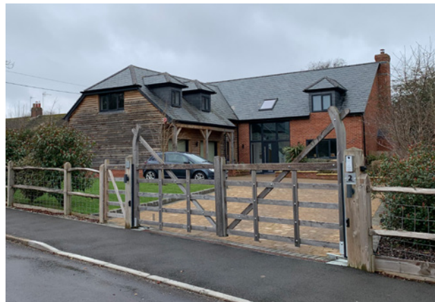
Figure 36: The use of hipped dormer, timber weatherboarding, slate and red brick on this contemporary property echos the historic material palette. The fencing reinforces the rural setting.
