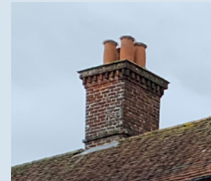
Masonry chimney stack
