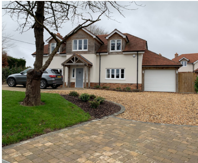
Figure 32: A recently constructed detached house with timber weatherboarding and rendered facade, as well as other features such as the porch and gabled dormers, which reflect the historic character of the village.
