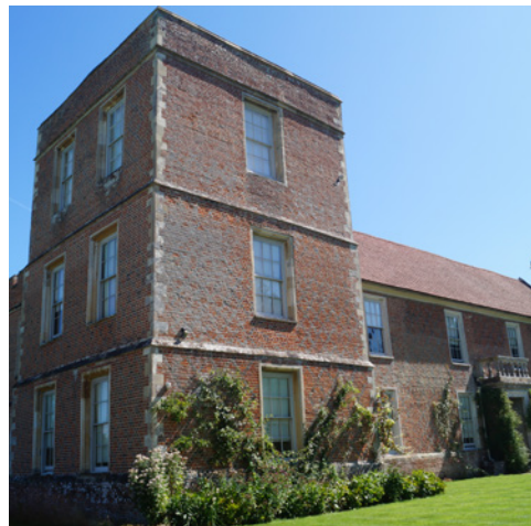
Figure 15: The Vyne, Grade I listed house
