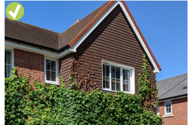
Figure 68: Example of a property with vegetation on the facade, elsewhere in UK
