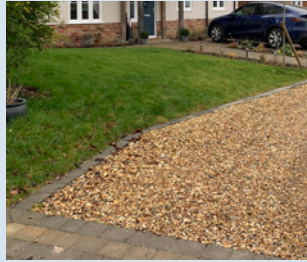
Gravel and block edging
