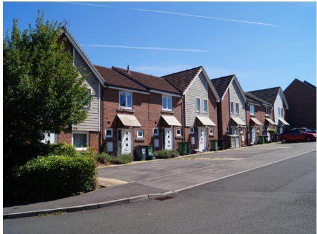
Figure 54: Terraced properties with a large area of car parking outside the houses and no green front garden.
