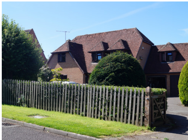
Figure 39: Two storey house with dormer windows and half-hipped pitched roof.
