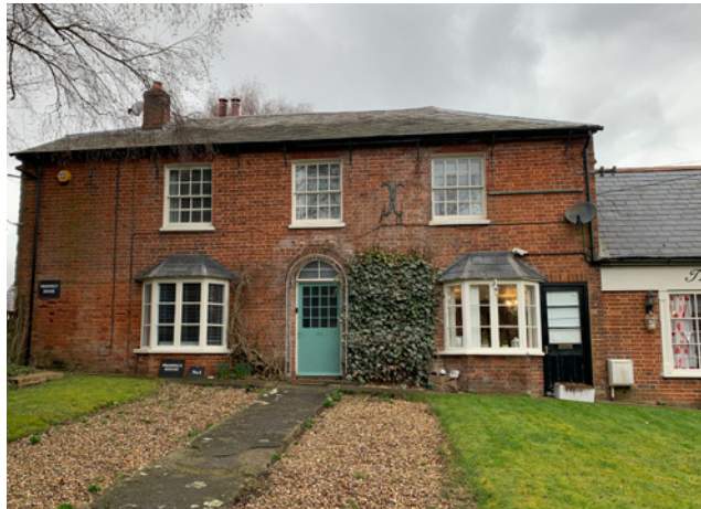
Figure 18: The Old bakery Emporium on Aldermaston Road, which features many positive Victorian details such as bay windows red clay tiles.
