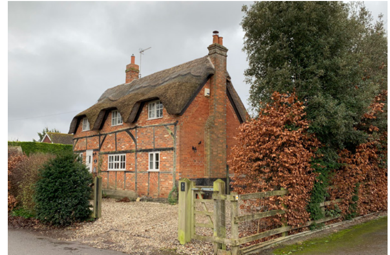
Figure 25: Swan Cottage, Kiln Road, is recognisable for its intricate and unique features (timber banding, red brick, thatched roof) is an important focal point in this CA and the wider village.
